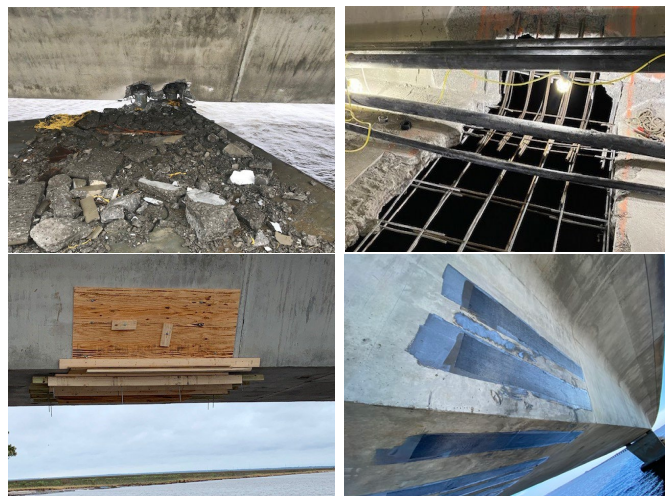
Figure 16: FRP repairs on Garcon Point Bridge in FL.
