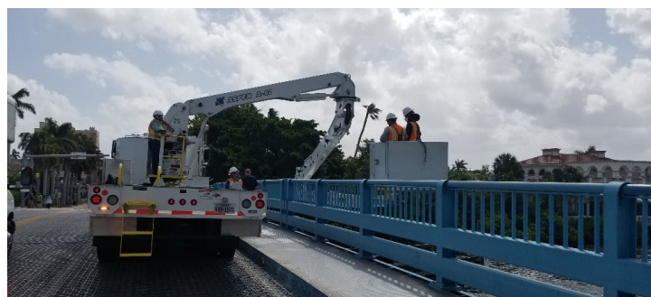
Figure 14: Our privately-owned Snoopers allow our teams to work above, below, or alongside structures safely, have a horizontal reach of 62 ft., and require no outriggers to operate.
